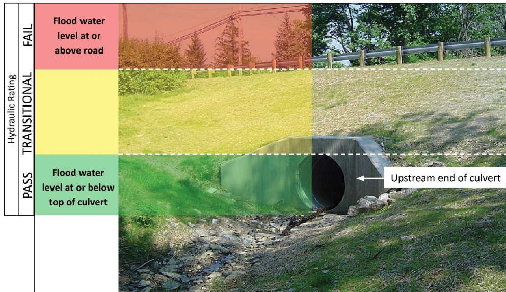
FIGURE 5: Example of how the hydraulic rating is applied to a culvert evaluation.
