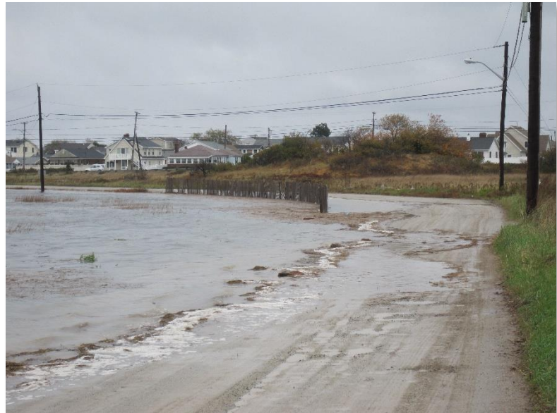
Figure 2. 2013 King Tide flooding at Cross Beach Road.
