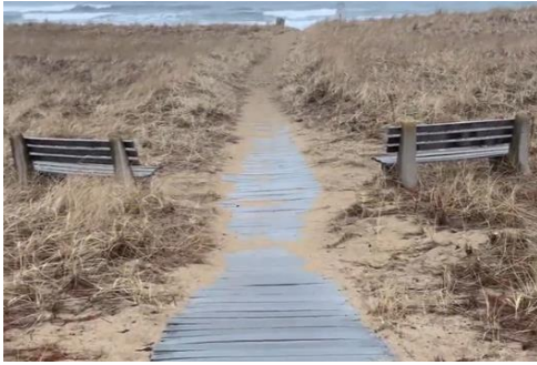
Figure 5: Bottom of walkway buried
