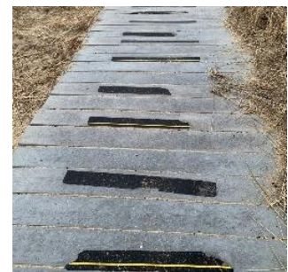
Figure 3. Previously installed slip resistant tape
