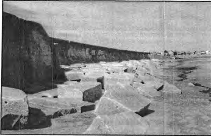
Seawall with stone revetment toe protection
