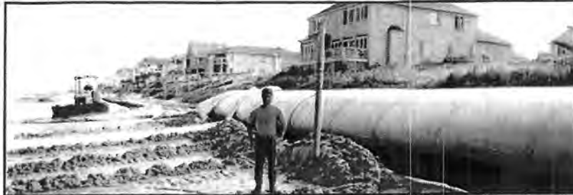
Sand filled geotube berm (Photo courtesy of Bradley Industrial Textiles, Inc.)
