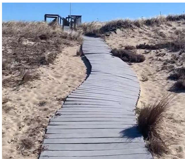
Figure 3: Shifting boardwalk foundation; bare areas of sand and footprints observed alongside the walkway; Chelmsford Street
