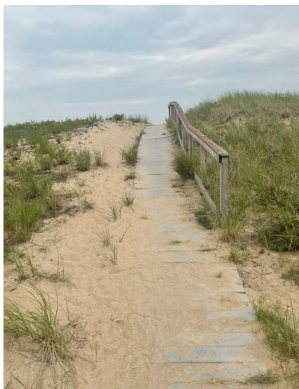
Figure 4: Sand accumulation on boardwalk, bare areas of sand and footprints observed alongside the walkway; Andover Street
