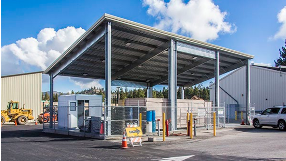
San Bernardino County, CA HHW Facility—this photo also shows prefabricated hazmat storage buildings under a roof structure.
