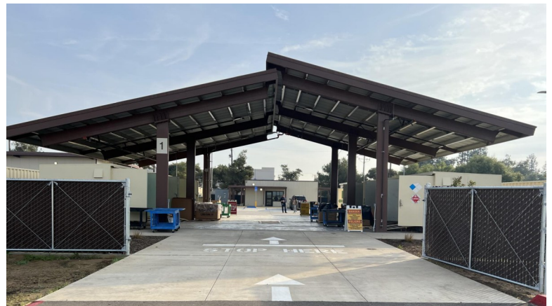
Fresno County, CA HHW Facility—this photo shows where cars enter the covered unloading area, carts used to unload vehicles, prefabricated hazmat storage buildings.
