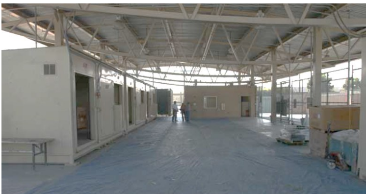
City of Los Angeles, CA—this photo shows prefabricated hazmat storage buildings, used for flammables and other high hazard materials, under a roof.
