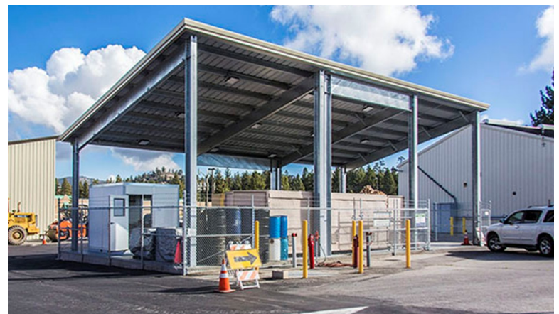
San Bernardino County, CA HHW Facility—this photo also shows prefabricated hazmat storage buildings under a roof structure.
