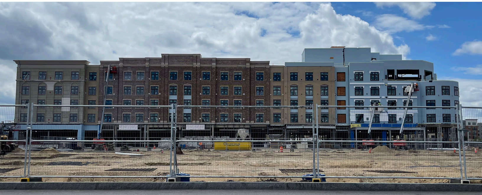
Multi-family housing under construction in Salem, NH, 2022.
